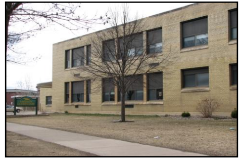
Emerson Elementary School
